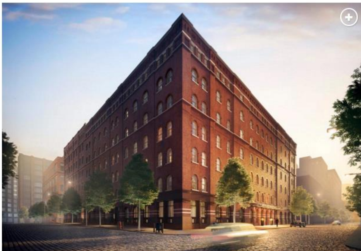
443 GREENWICH: One of the last untouched warehouses in Tribeca, 443 Greenwich has now been transformed into 53 condos, but its original 1880s girders and columns (below) serve as visible reminders of its past life.
